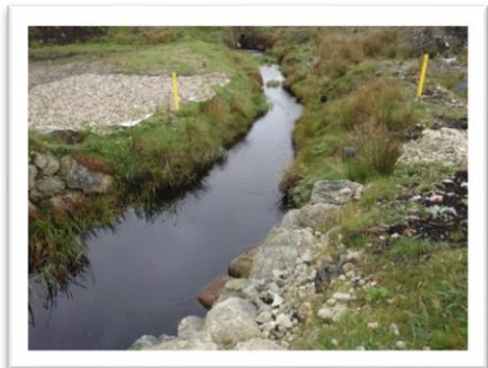
Photo OW1-3 shows silt trap on the left bank.
