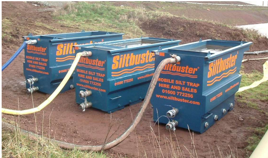
Figure 5.3 Temporary site settlement tanks (Source: Siltbuster)
